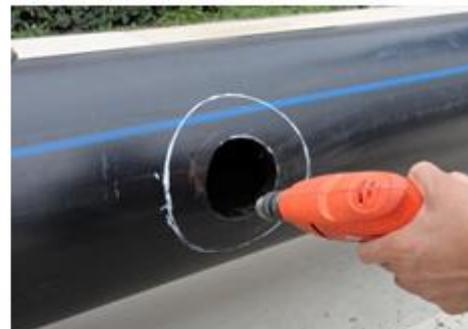
3.3 Scrap the fusion zone marked ( The whole saddle bottom part area)
